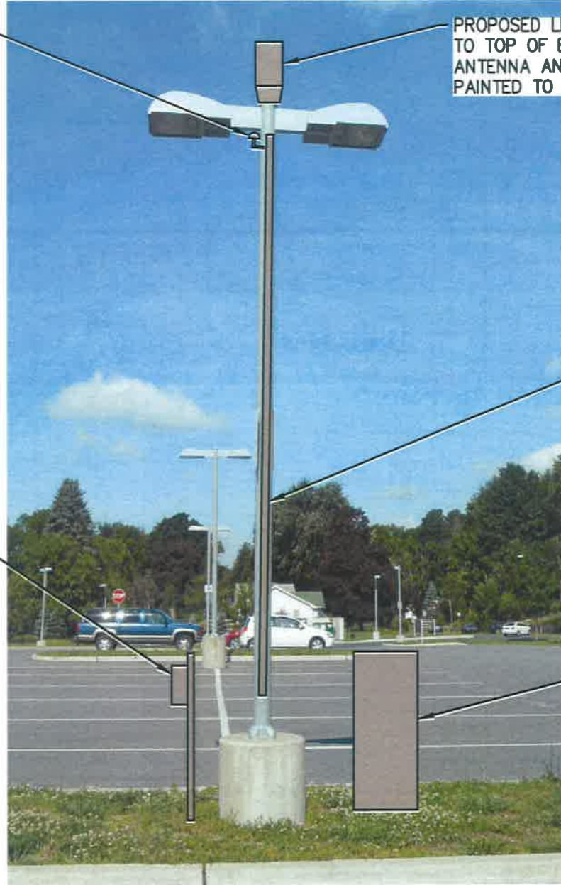
PROPOSED CHARLES CABINET MOUNTED AT EXISTING LIGHT POLE
