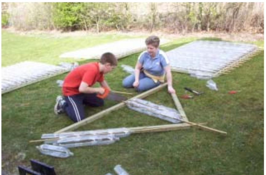
Screw the triangular gables to the posts and include a top beam and vertical supports (from the top of the gables to the top of the front and back panels). The sloping sides of the roof can be made out of similar panels as the walls. These can then be screwed onto the top beam, gable ends and top of the side panels.
