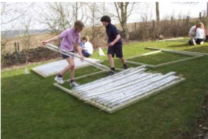
Place the bottles and canes onto the frames to be attached at the top and bottom of the frame.
