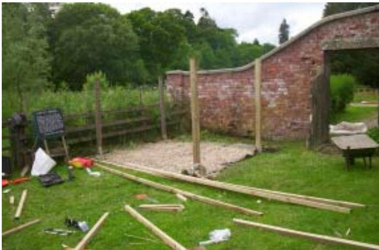
3. Fix 4 posts vertically into the ground. Treated 4" x 4" posts cemented a couple of feet into the ground works great. These are for the corners of the greenhouse. Put slabs or mulch around and inside to suppress weeds.
