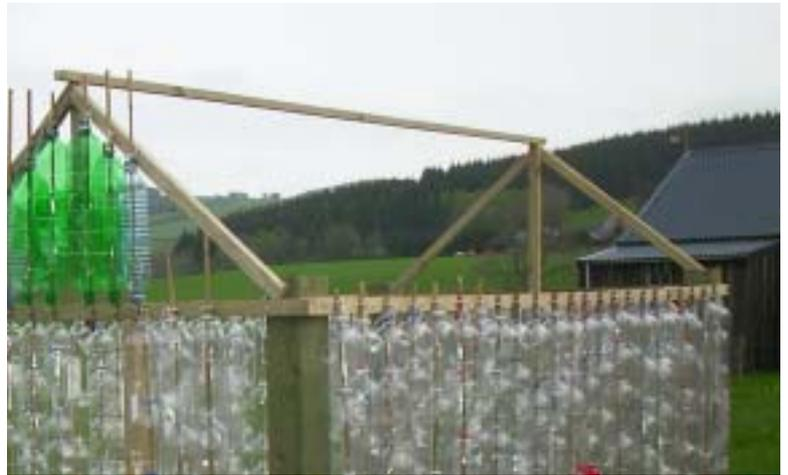
The door can be made of a smaller frame hinged to a larger frame making up the front wall. Make the door smaller than the inside of the frame to allow it to open freely even if it sags.
